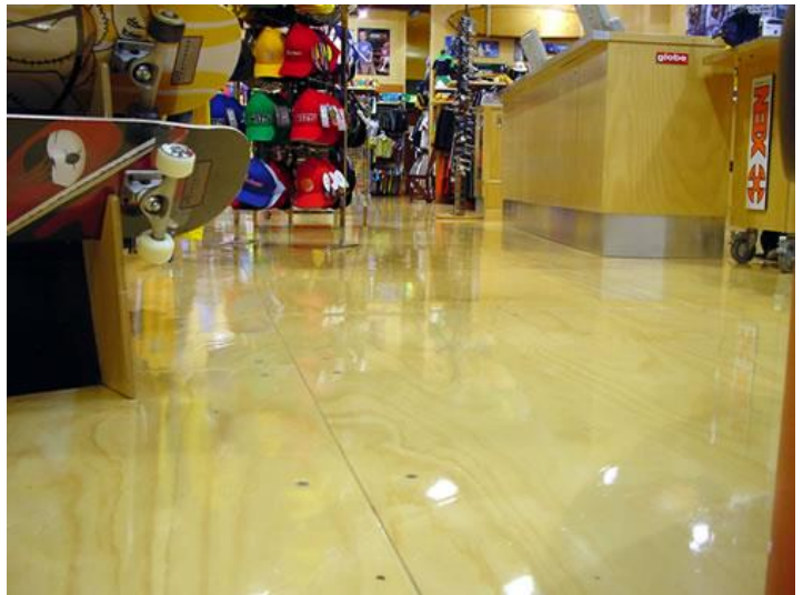
Structural Plywood Flooring, Clear Finished, Shop Floor
